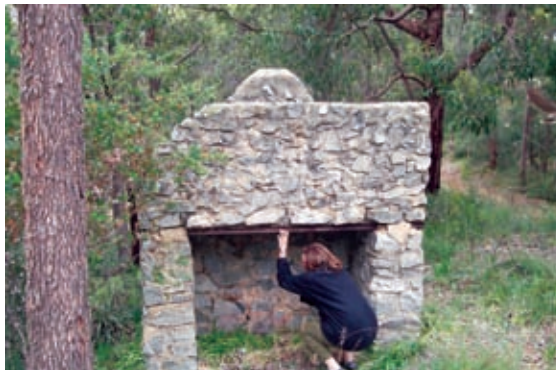
Above: The stone fireplace on Peet road was built by the sustenance crews building the channel to dry their clothes and keep warm in the chilli mornings of winter.
